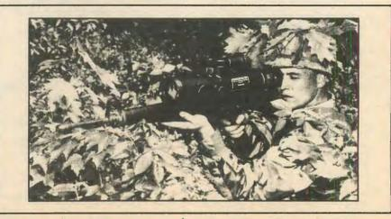
Some first generation, cascade type image intensifiers are still used in the field. This AN/PVS-2 was developed in the late 1960s and was advanced compared to other first generation designs.
